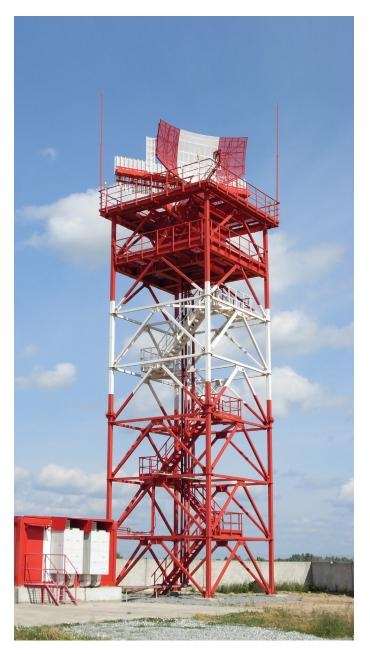
**Antenna system** shapes a dual-beam antenna pattern. The MSSR antenna is installed on the support and rotation device together with the PSR antenna in "back-to-back" position.
