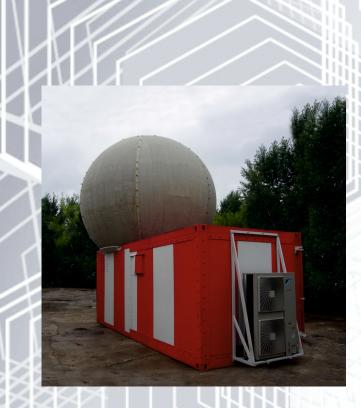
Terminal Area Radar Complex "RC-10RA" intended for regional airports has primary surveillance channel of S-band and secondary surveillance channel of RBS mode, complies fully with the requirements of international standards, the standards of the Russian Federation and Russian Federal Aviation Regulations.
